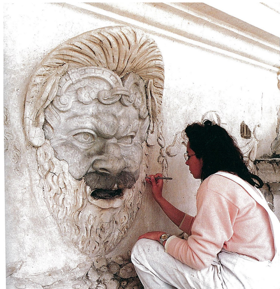
Theatrical mask, currently being restored, central section of the façade of the Villa Medici gardens in Rome. Final cleaning phase. Ph. SEI.
